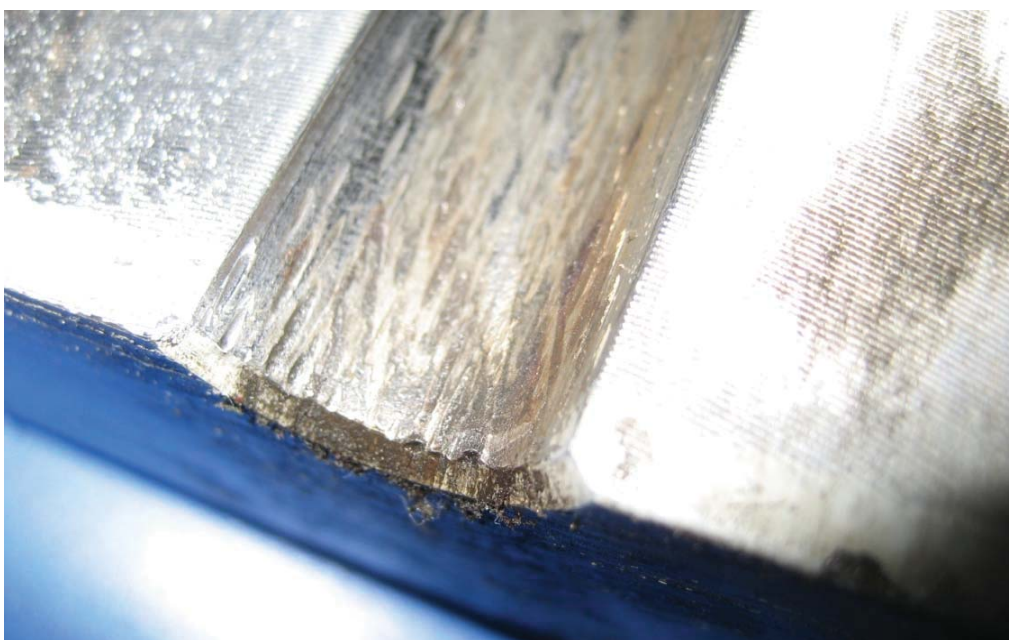
Figure 12: Typical condition of the clamp groove at the exit points after the fatigue test (FLC02).
